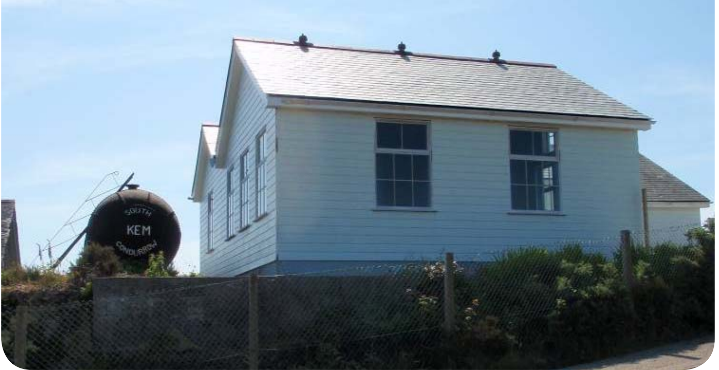
New winder/ compressor house at King Edward Mine funded by DtE (Image: Ainsley Cocks)
